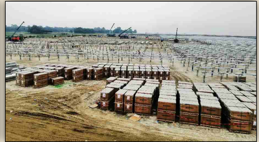
MMS Installation and plant storage
