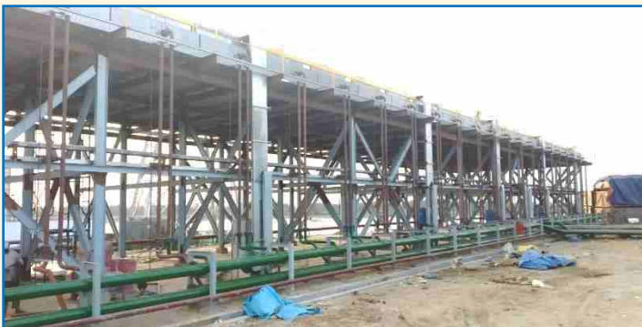
Radiation structure Construction
