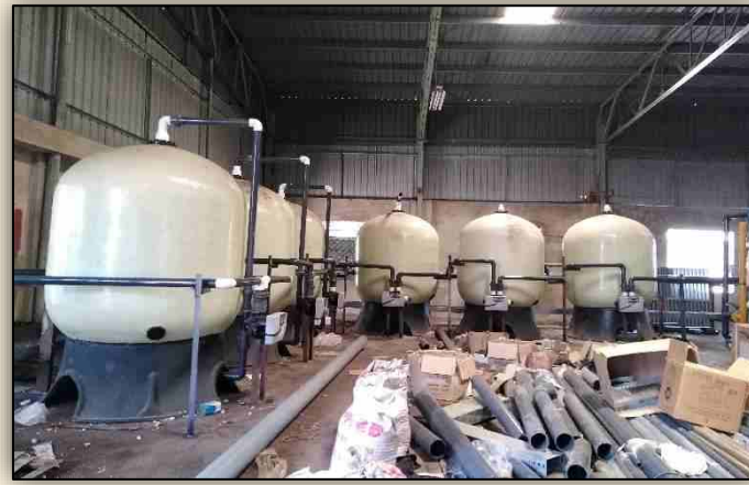
WTP - 75M 3 /Hr Capacity (TK GROUP, Chittagong)
