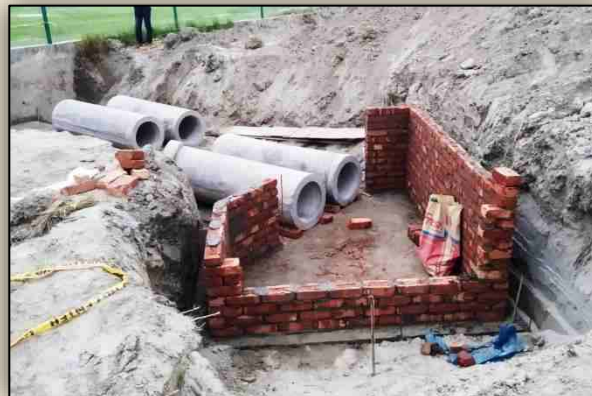
Plant Drainage system Construction
