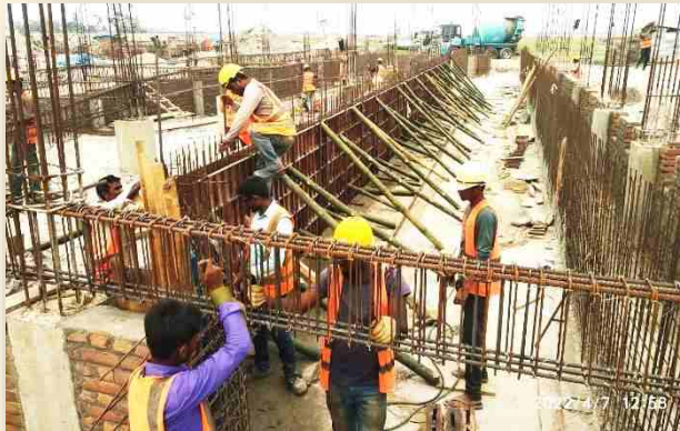
Main Control Room (Construction)
