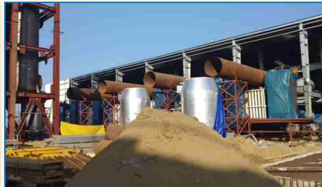
Exhaust duct Construction
