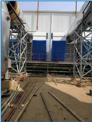
Charge air filter platform Installation
