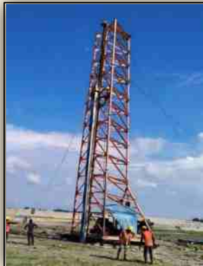
Precast pile drive
