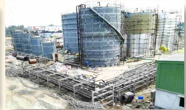
Pipe Const. & Tank Insulation
