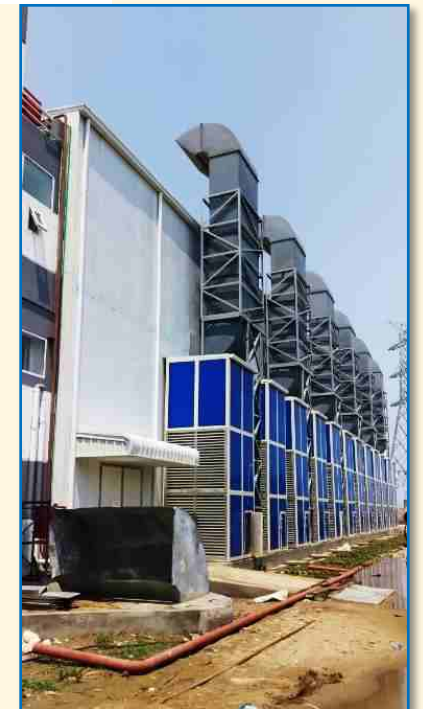
Alternator duct Construction
