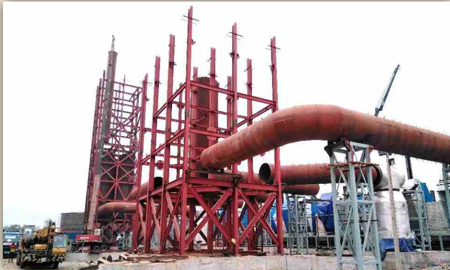
Stack Tower Construction
