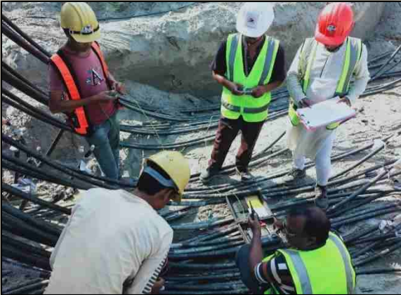
Cable Schedule work
