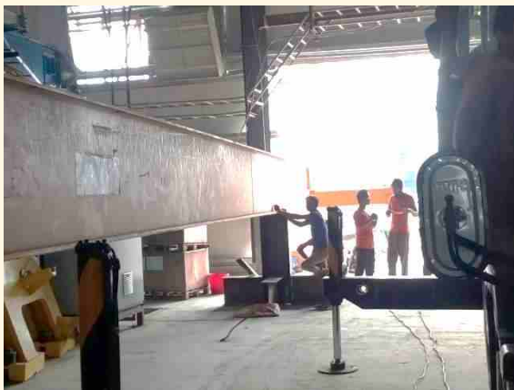
Over Head Crane Installation
