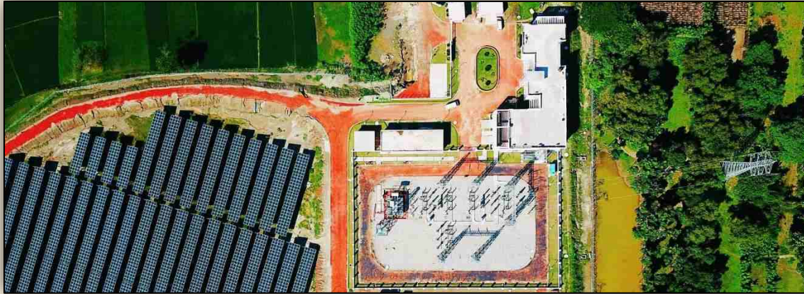
Substation, Admin and Control building
