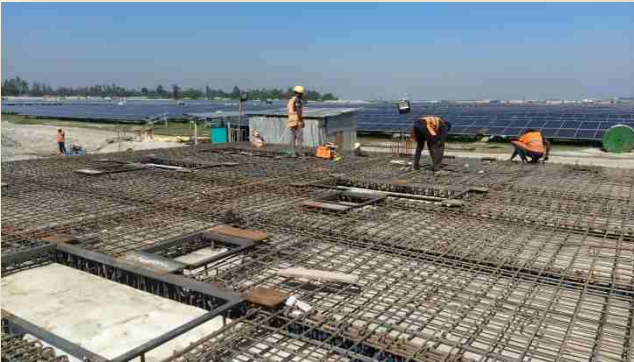
ICR Rebar Work
