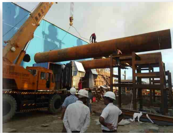
Engine Exhaust Gas Duct Construction
