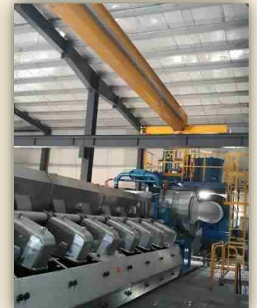
Over Head Crane Installation
