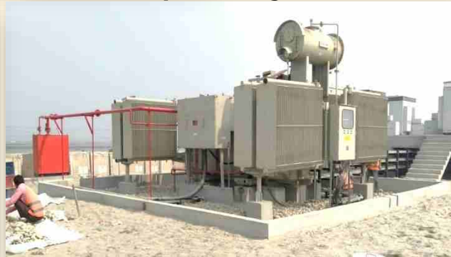
IDT after Installation
