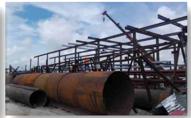
Radiator Structure Installation
