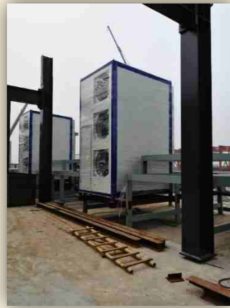
Ventilation System Installation
