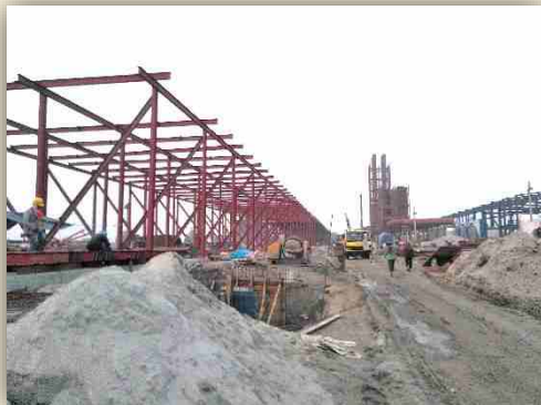
Radiator Structure Construction
