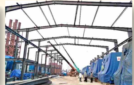
Engine Hall Construction
