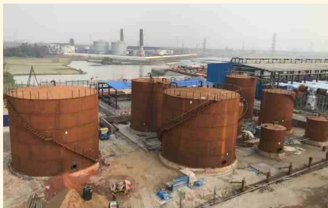
Tank Under Construction
