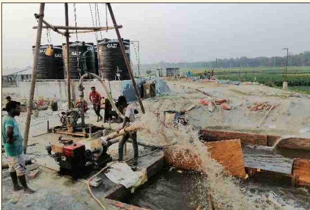
Module Cleaning system and Deep Tube-well Installation
