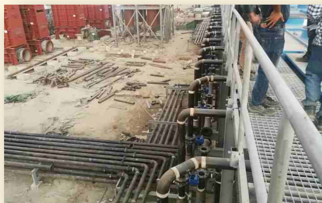
Pipe Line Installation
