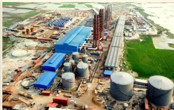
Plant Under Construction
