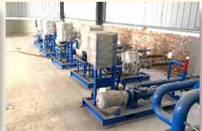
Fuel Treatment Plant Installation
