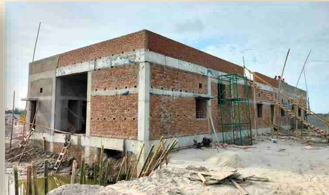
Main Control Room (Construction)
