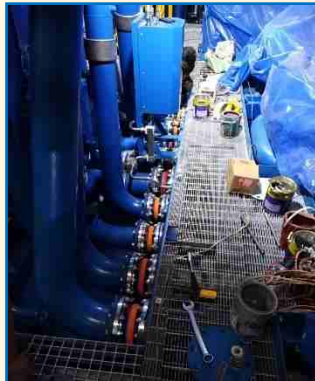
Module Installation at Engine hall
