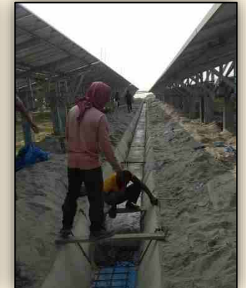
Drainage slab construction
