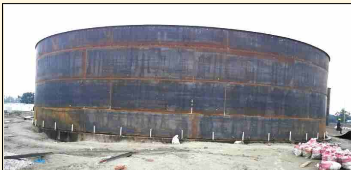
TANK UNDER CONSTRUCTION
