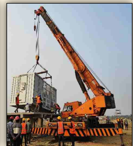
Inverter Installation
