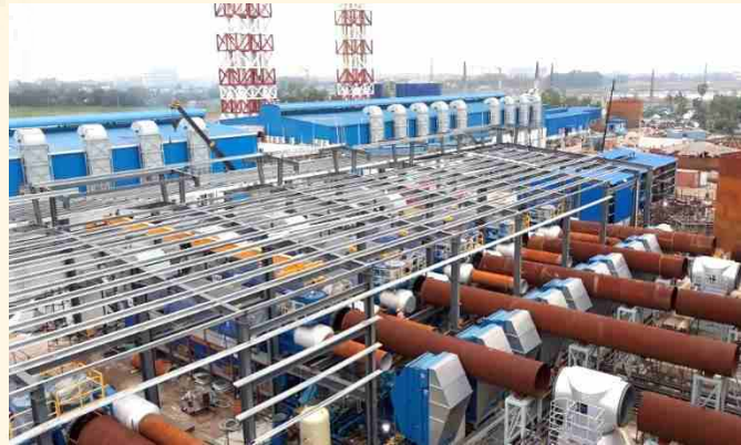
Engine Hall Construction
