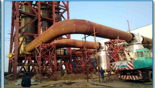
Exhaust duct Construction
