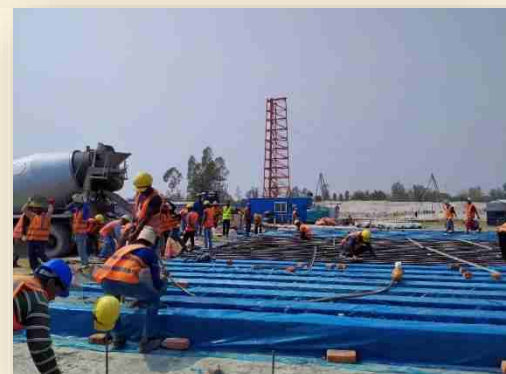
13m Pile Construction
