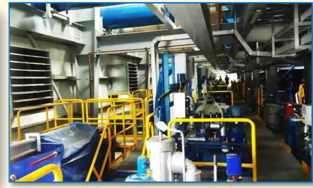
Module Platform Installation
