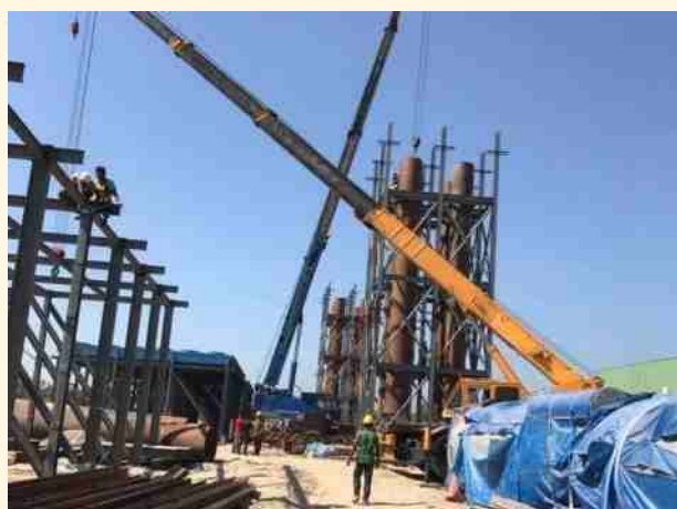
Stack- Radiator structure Installation
