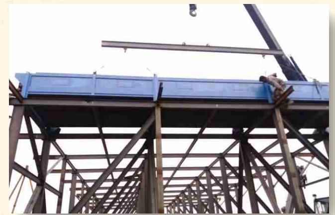
Radiator Installation
