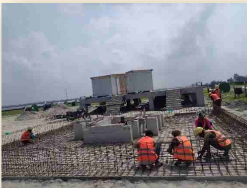
IDT Rebar work
