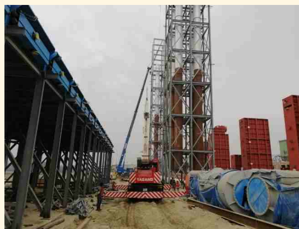
Stack- Radiator structure Installation
