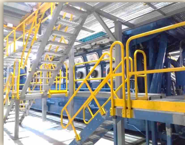
Engine Maintenance Platform
