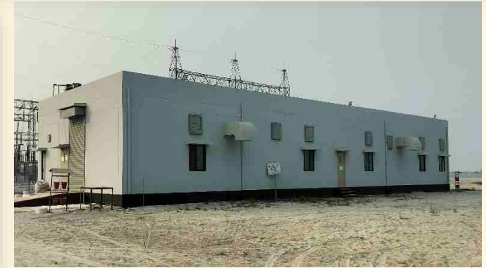
Main Control Room
