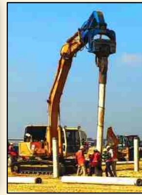
LHV pile Drive
