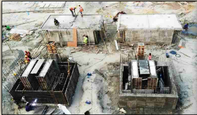
Substation Foundation Construction
