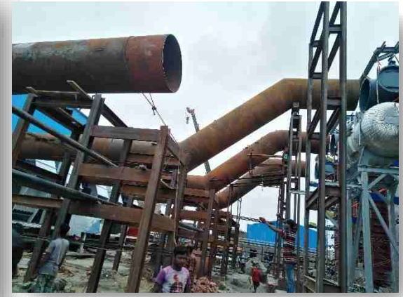
Engine Exhaust Gas Duct Construction
