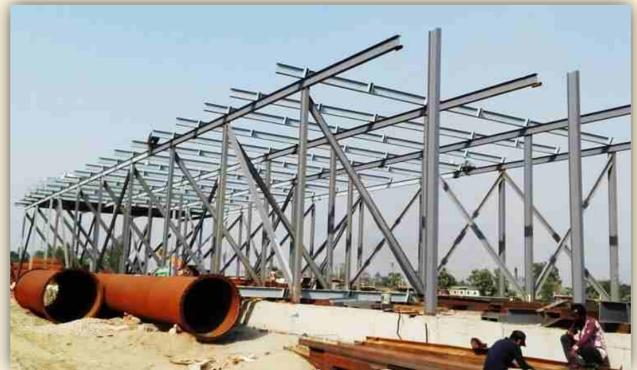
Radiator Structure Installation
