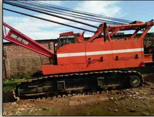
Crawler Crane 80T
