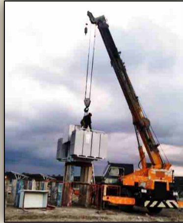
Transformer Installation
