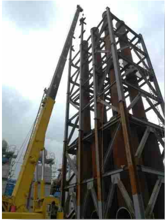
Stack Tower Construction
