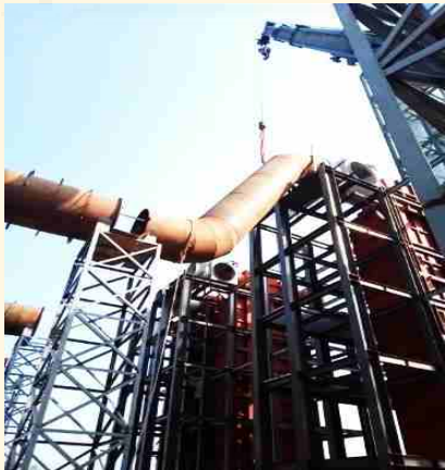
Exhaust duct & support Construction
