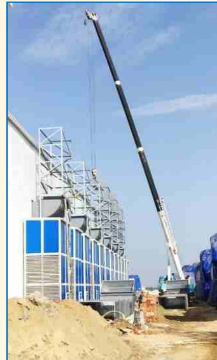
Alternator duct Construction
