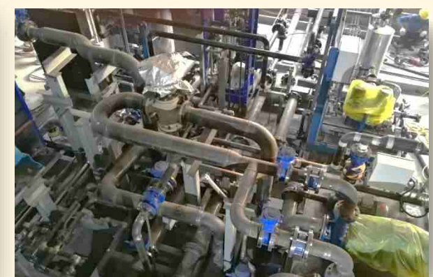
Pipe line Installation
