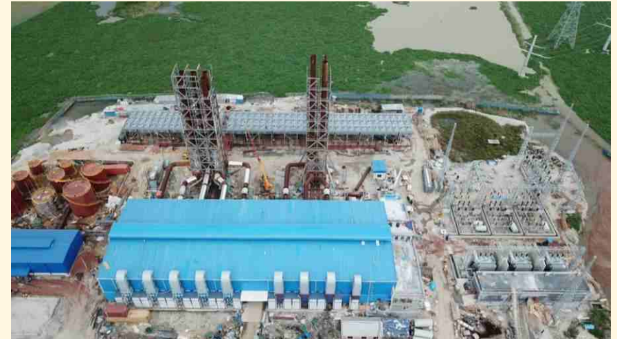
Plant Under Construction
