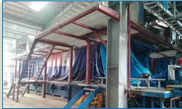
Engine Hall Maintenance Platform Construction
