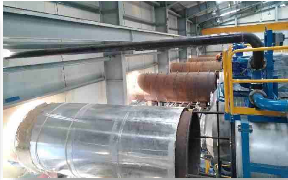
Exhaust Duct Alignment
