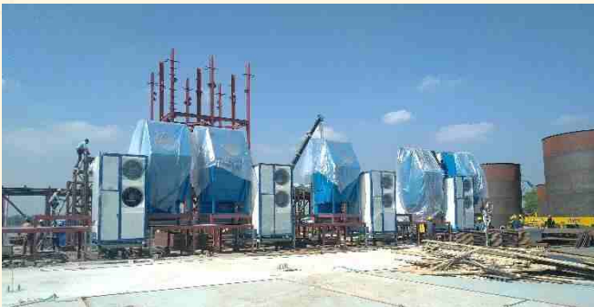
Ventilation System Installation
