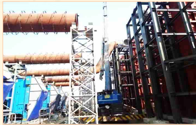
Exhaust duct & support Construction
