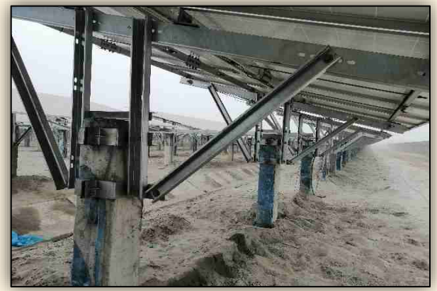
MMS and PV panel Installation
