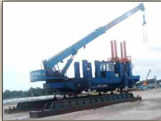
Hydraulic Pile Drive
