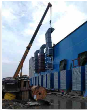
Alternator Duct Const.
