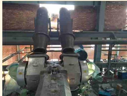
Charge air duct Installation
